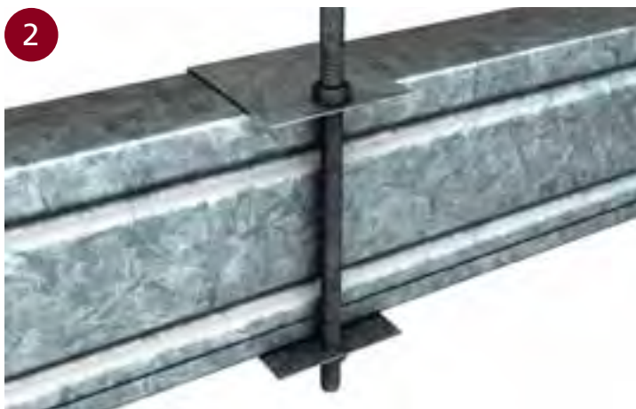
■ ATTACHING STUDS TO THE ROD
